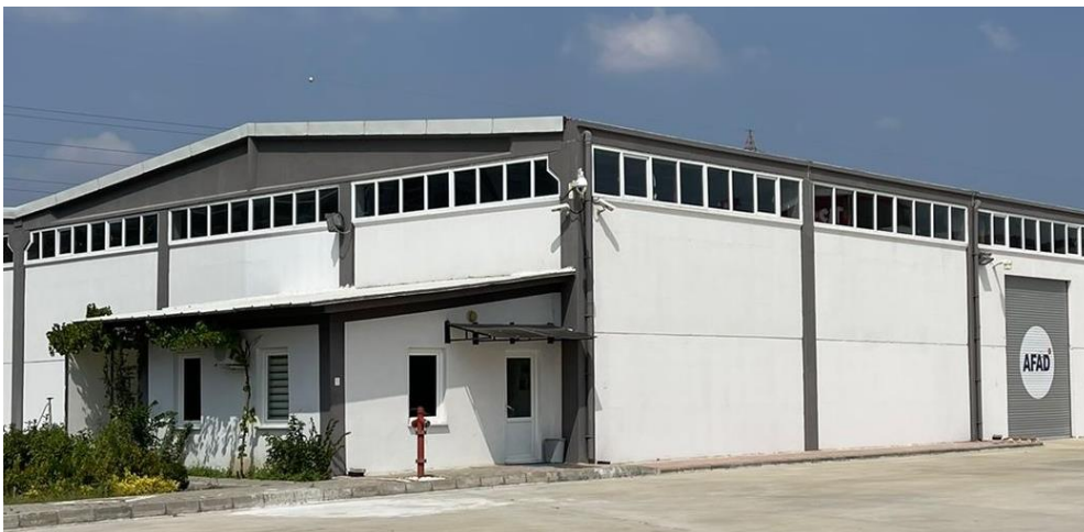
Figure 4. Logistics Warehouse of AFAD in South Marmara Region
